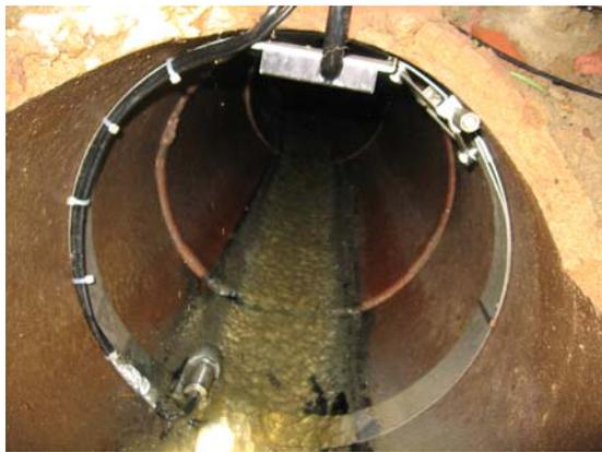
The upper sections of the collection system presented a different challenge. Shallow flows were such that the velocity and pressure sensors remain out of the flow during periods of low flows as illustrated in the picture to the left.
